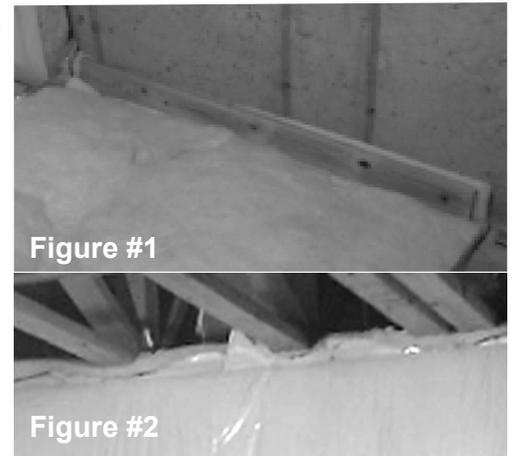
details. Trim any excess insulation for a neat appearance. Pull the release paper from the factory applied double stick tape. Overlap this 6" facing tab and adhere to the adjacent blanket.
